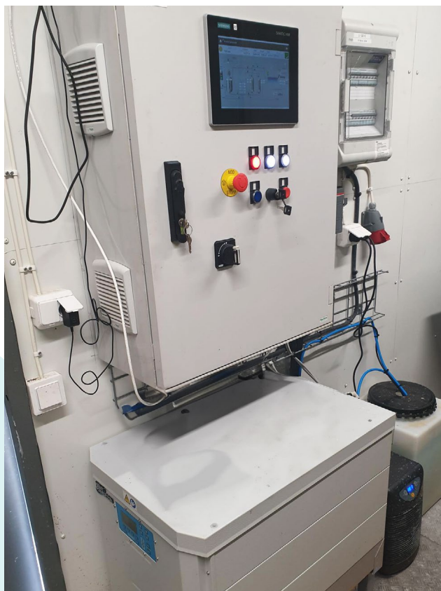
The AxoPur rectifier features a polarity switch that enables regular polarity shifts, ensuring optimal electrode performance and sustained energy efficiency.
