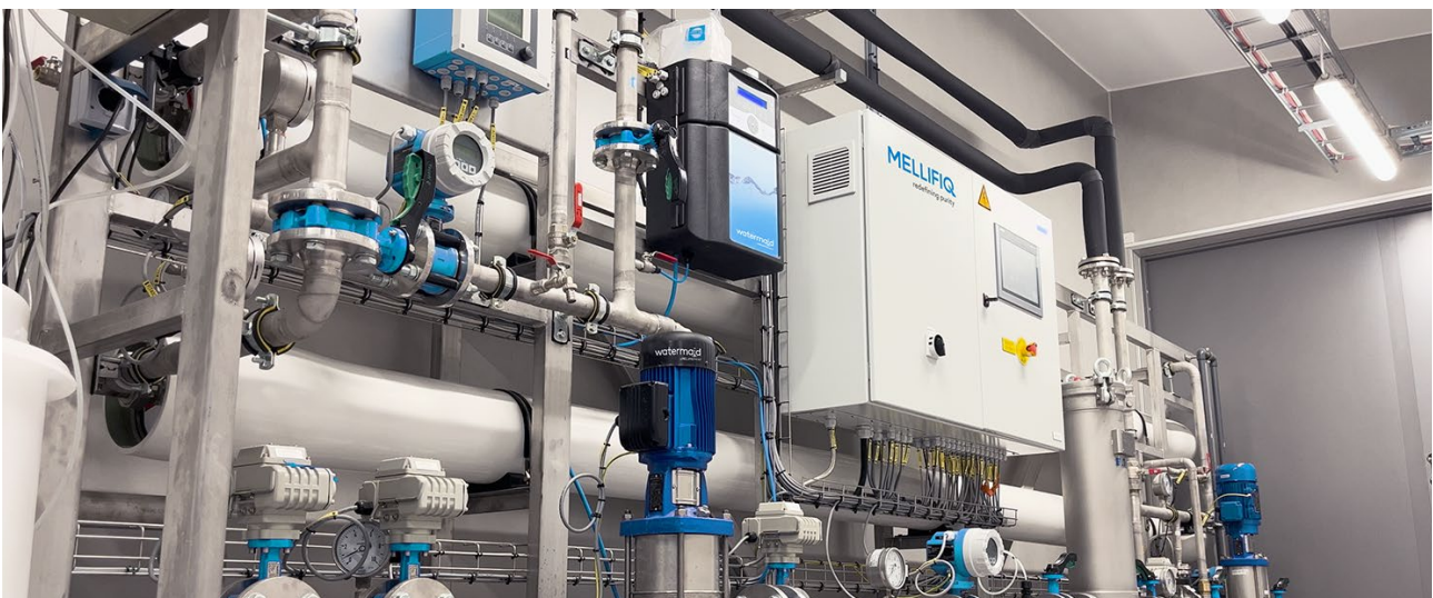
Finished installation of Water Maid CoraLuxe B2-N system for drinking water up to 9 m³/h permeate flow.
