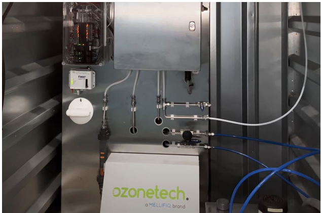
The RENA Pro B ozone system generates ozone for the treatment process.
