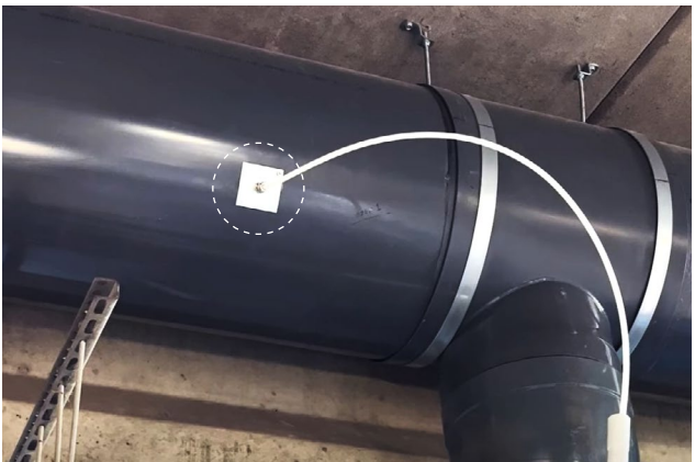
The exhaust gas stream flows through merged air ducts, where ozone is injected to react with VOCs.
