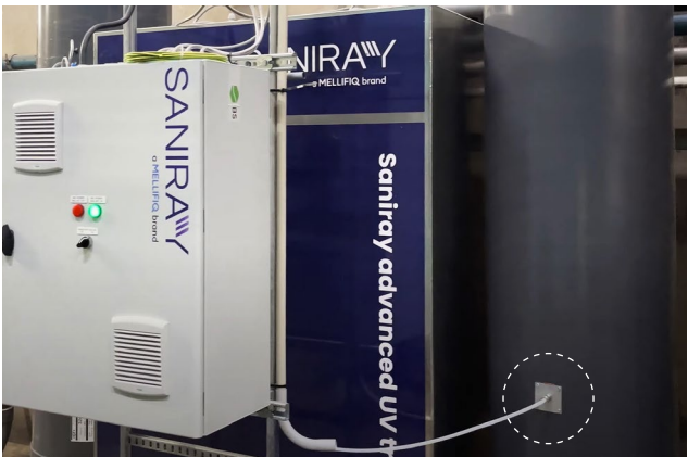
Saniray advanced UV-C technology enhancing ozone-VOC reactions to break down challenging VOC compounds.
