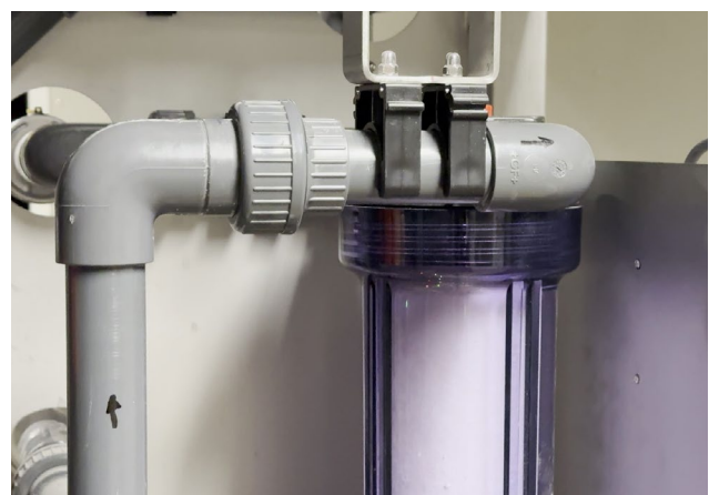
The stations are equipped with a cartridge filter, fan, permeate pump, backwash pump, and electronic meters for flow, turbidity, and temperature.
