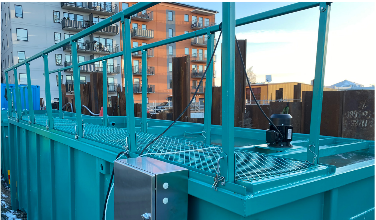
The two AquaFloc containers, each measuring 20 ft, are particle separation systems that remediate groundwater using flocculation processes.
