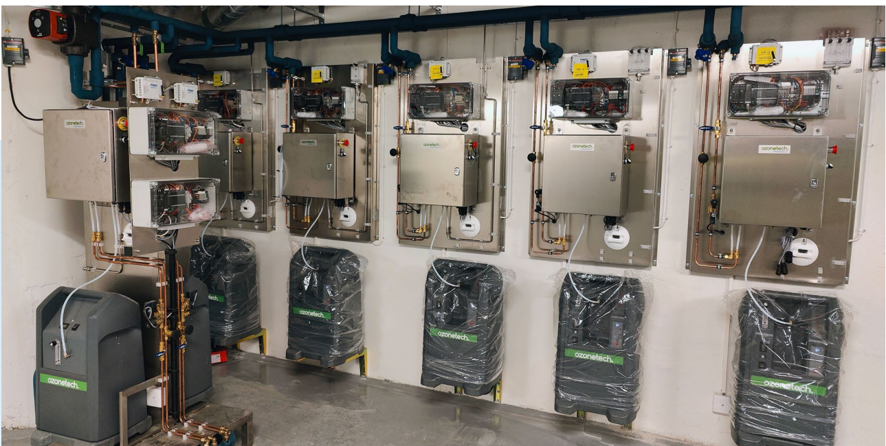
The RENA Kitchen Solutions units are installed in the garage beneath the restaurant, managing all kitchen exhaust air from a single location.
