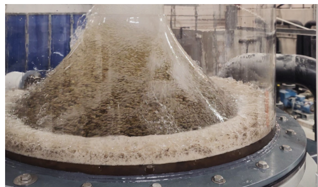
Ozone injection generates microbubbles that coagulate and physically separate dissolved organic matter.
