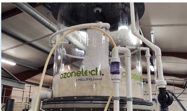
Fractionators are essential tools in applications where effluent water contains large organic particles, commonly in aquaculture, zoos, and aquariums.
