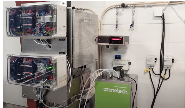
The installation includes an ozone generator and cooling system, along with an ozone meter, sensors, and the O3Eye™ control system to monitor and report the status of the ozone generators.
