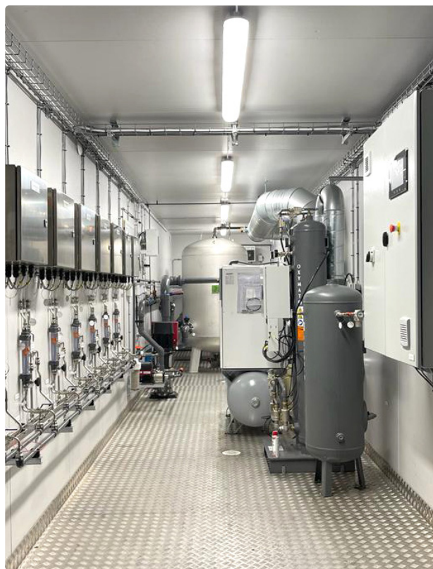
A fully containerized advanced water treatment system featuring WaterMaid FlexKarb and Ozonotech RENA Vivo technologies.
