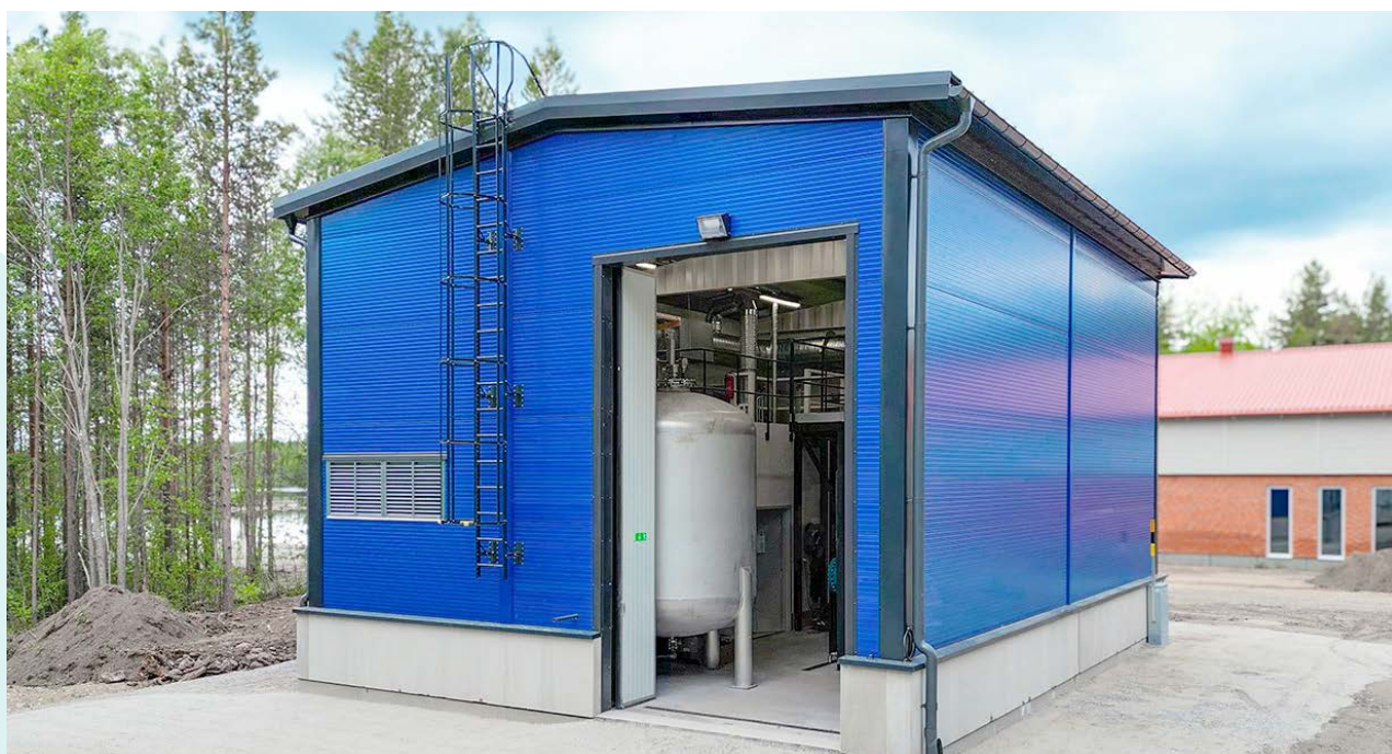
A fully equipped water treatment facility designed to remove pharmaceutical residues.
