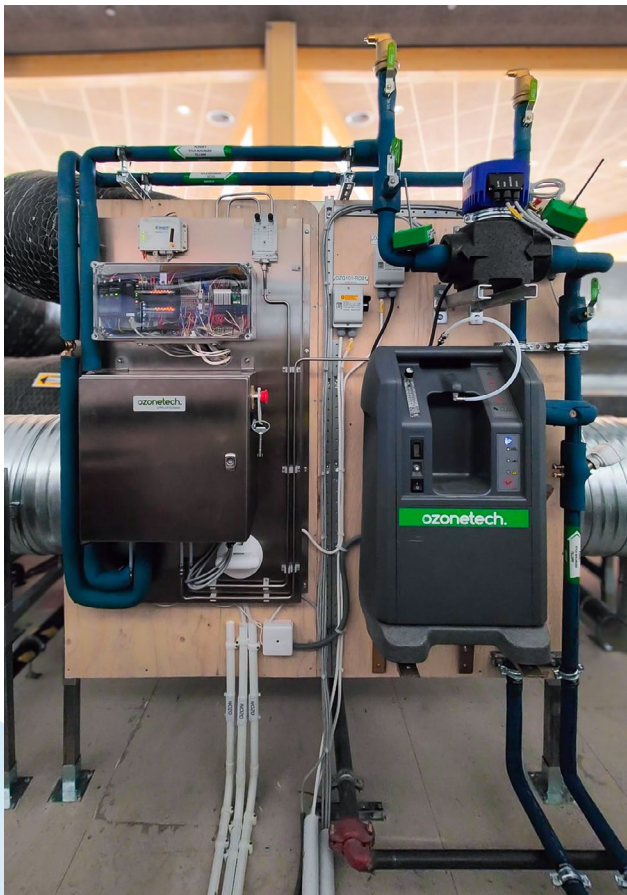
Mellifiq's RENA Kitchen Solution installed at Terminal 5, Arlanda Airport — utilizing advanced ozone technology to improve fire safety, odor control, and energy efficiency in high-demand commercial kitchen environments.
