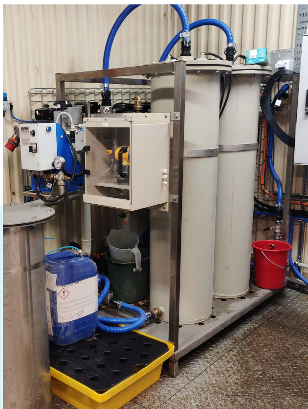
The solution included AxoPur reactors, a flotation unit and an intermediate tank, seamlessly integrated into the existing building.
