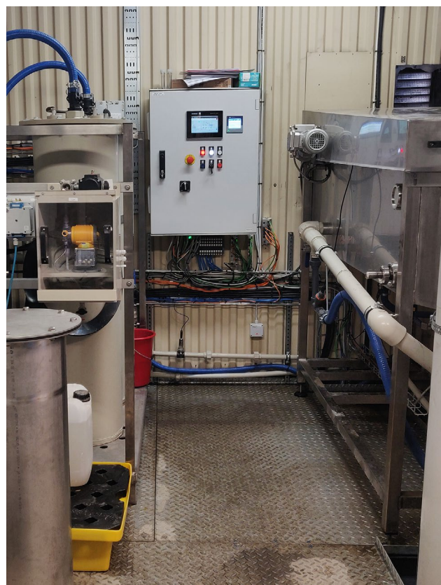
The solution included AxoPur reactors, a flotation unit and an intermediate tank, seamlessly integrated into the existing building.
