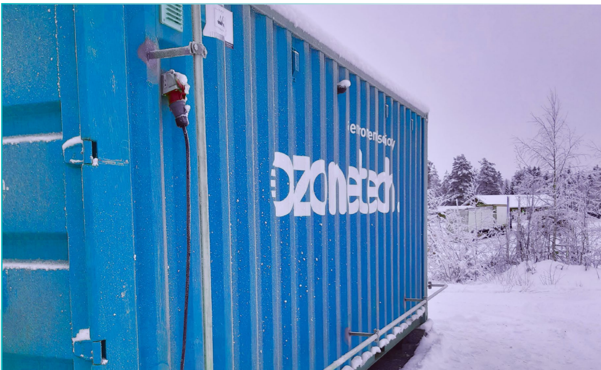
Exterior view of the containerized plant extension.
