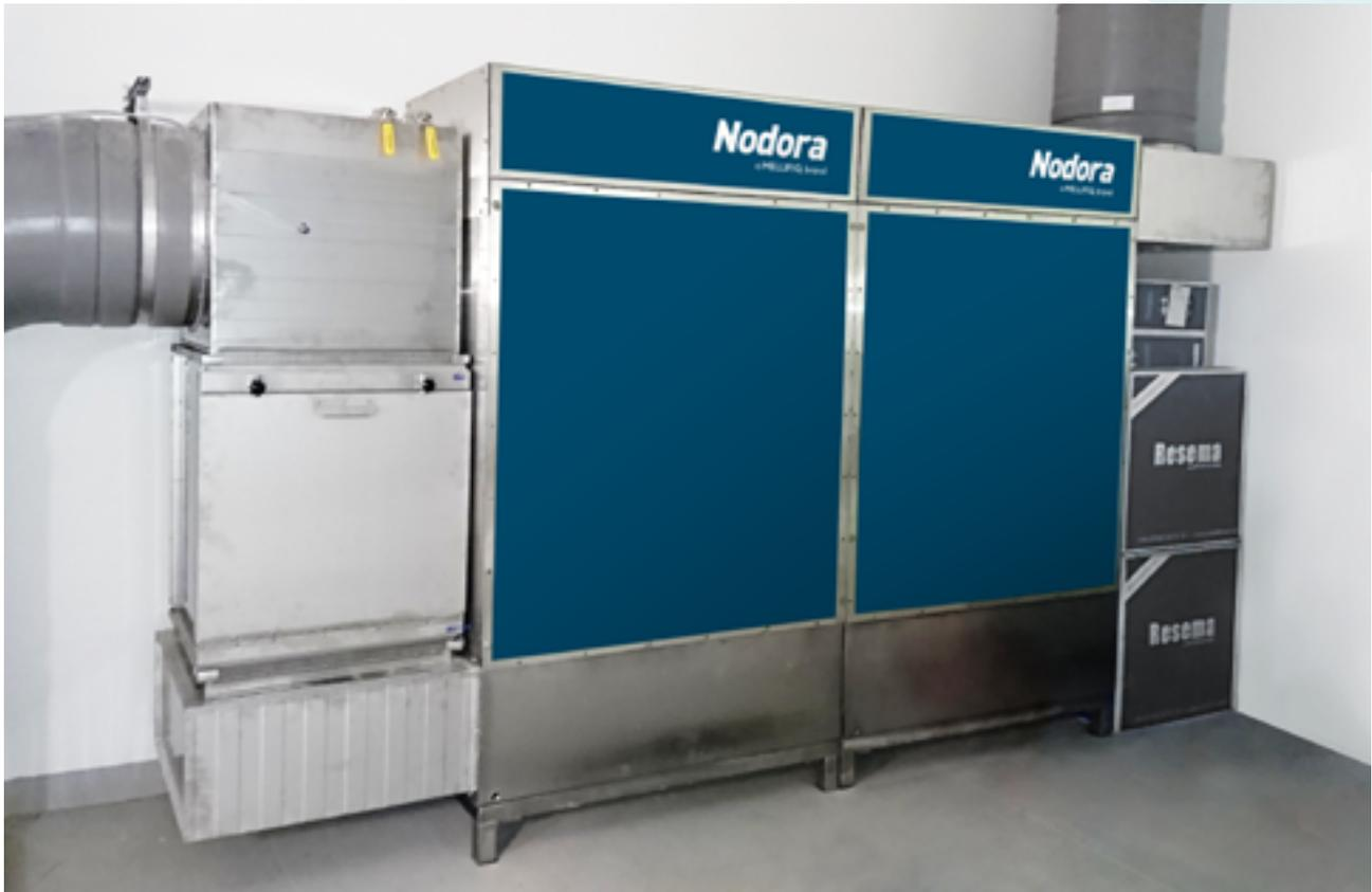
*The first treatment step consists of two Nodora Cat modules tailored to remove high H<sub>2</sub>S concentrations.*
