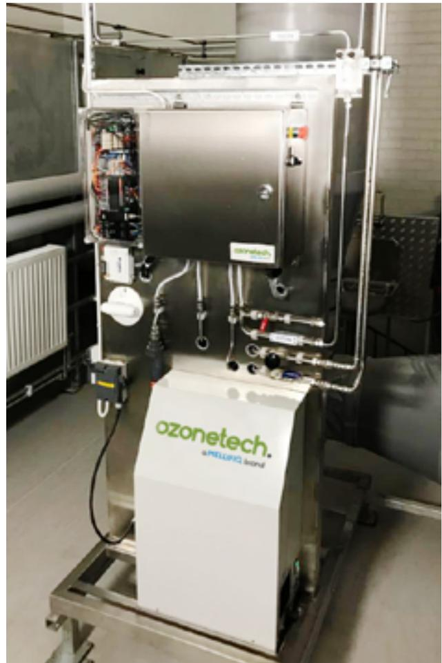
*The three RENA Pro systems produces the ozone volumes and concentrations necessary to eliminate the remaining odors after the Nodora Cat treatment.*
