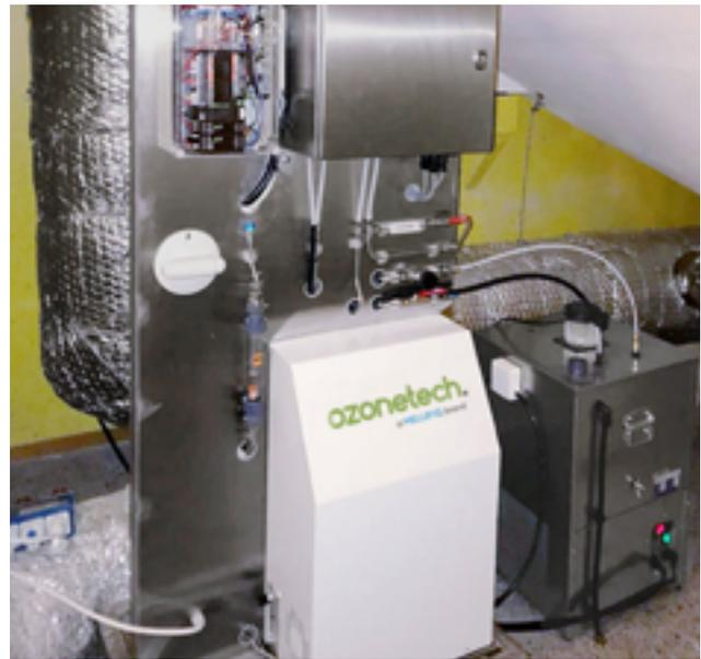
*The Ozonotech RENA Pro is skid-mounted and installed close to the ventilation duct where the ozone is injected. The operation is automatic and the installation includes closed-loop cooling system, oxygen concentrator, ozone sensors and remote monitoring.*
